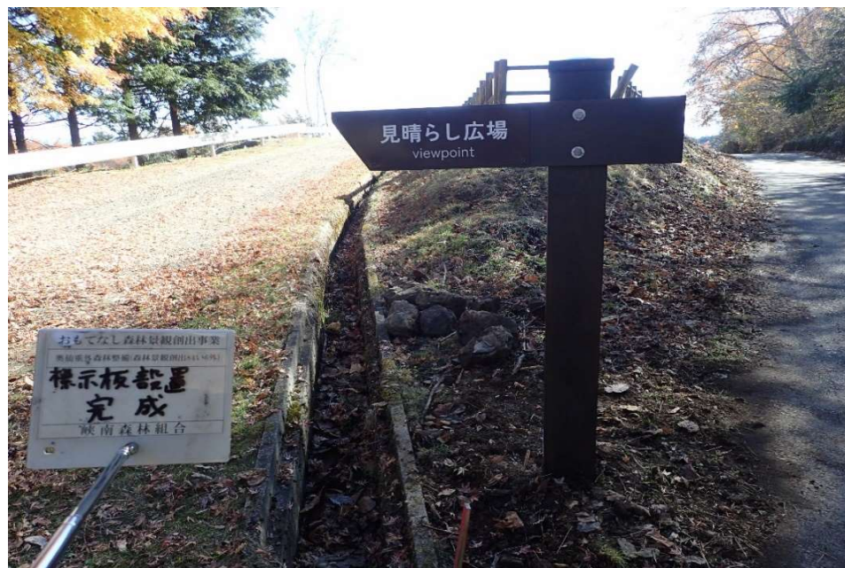
④ NO.1誘導標識板設置状況
