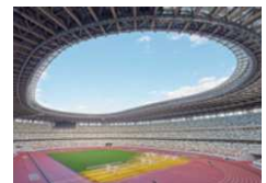
Forest Stewardship Council (FSC) certified larch timber from Yamanashi Prefecture used in the large roof structure above spectator seating in the Japan National Stadium.(Photo courtesy of the Japan Sport Council)
